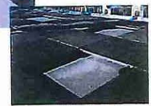
PORCELAIN PLANK ROOF PAVING BY TILE TECH
