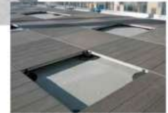
PORCELAIN PLANK ROOF PAVING BY TILE TECH
