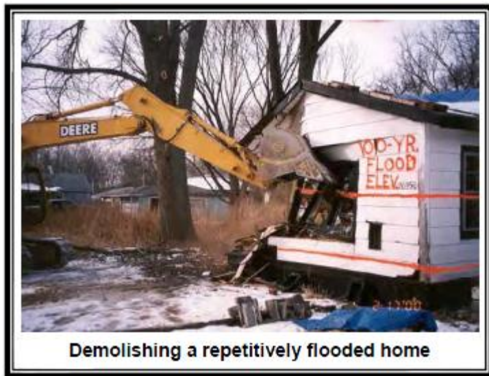
Figure C-5 Demolition of Flooded Home
