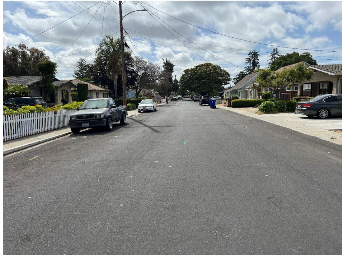
Figure 10: Arden Street After Patch Paving and Application of Rubberized Cape Seal
