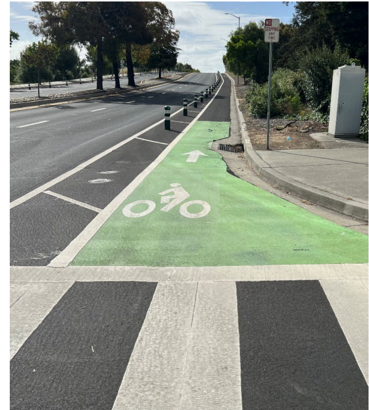
Figure 6: Newark Boulevard at Civic Terrace Avenue After Installation of New Class IV Separated Bikeway, Bike Lane Symbol With Green Thermoplastic and High Visibility Ladder Crosswalk
