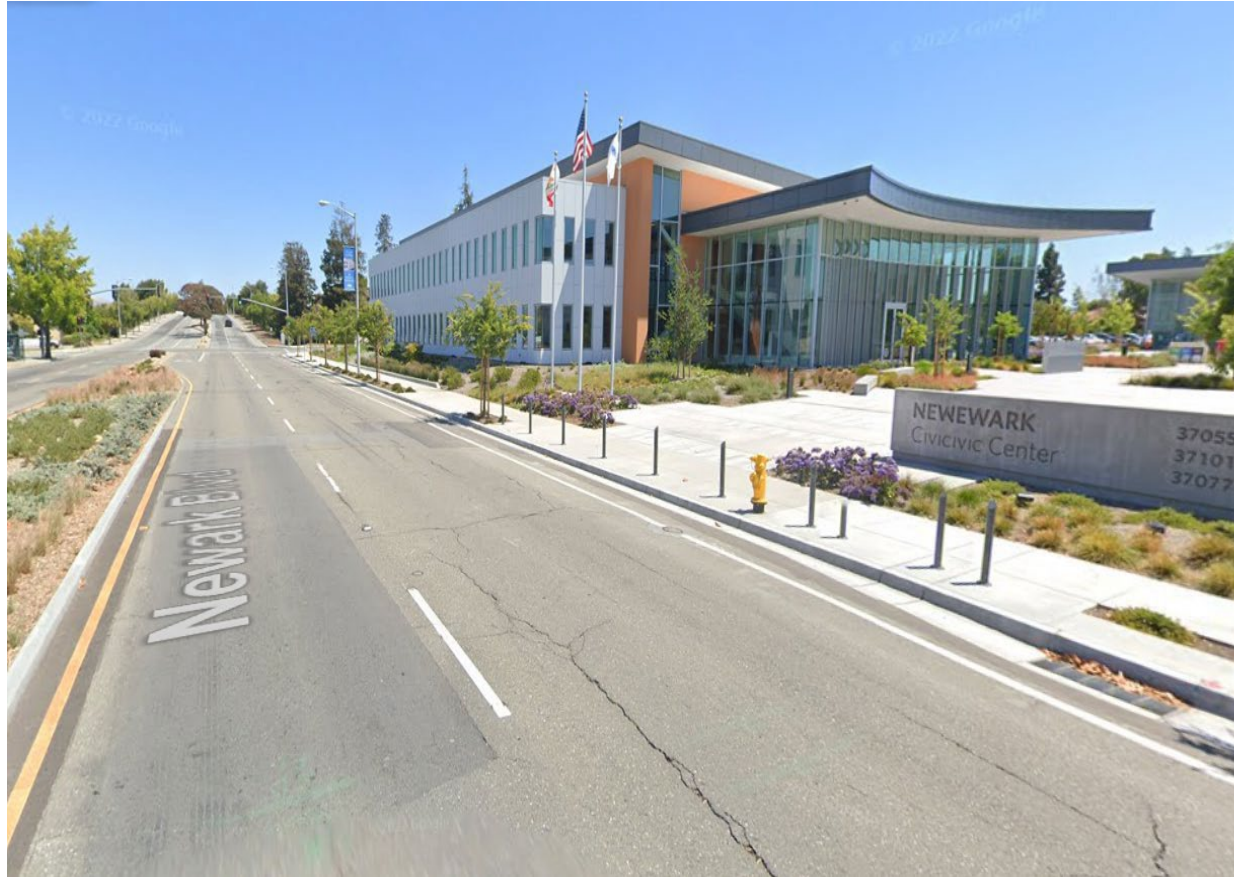
Figure 3: Newark Boulevard in Front of City Hall and Library (Before)
