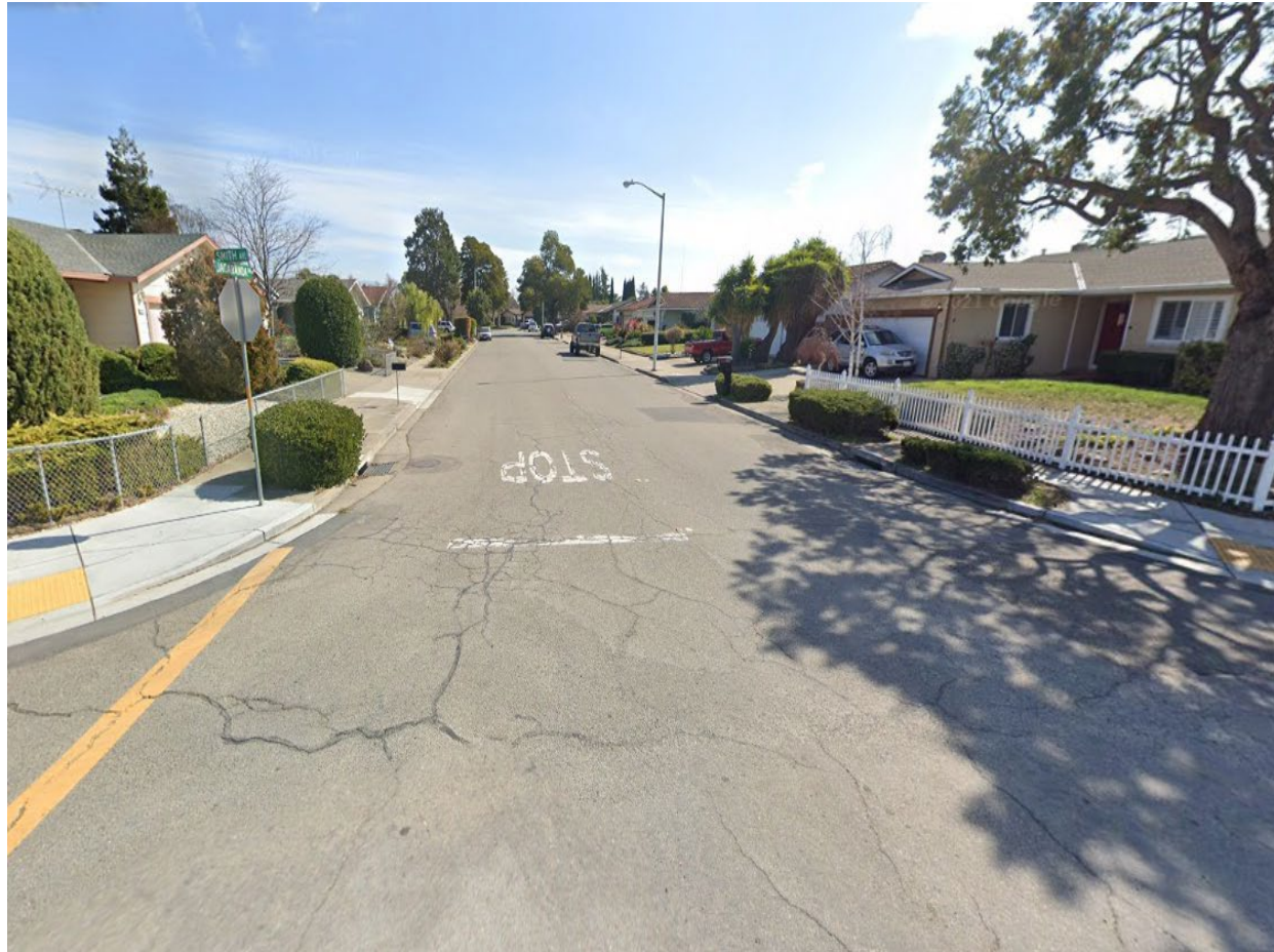
Figure 11: Jacaranda Drive (Before)
