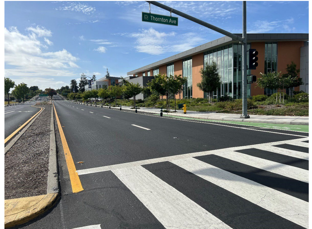
Figure 2: Newark Boulevard at Thornton Avenue After Patch Paving, Application of Slurry Seal, New Lane Striping, Class IV Separated Bikeway, and High Visibility Ladder Crosswalk
