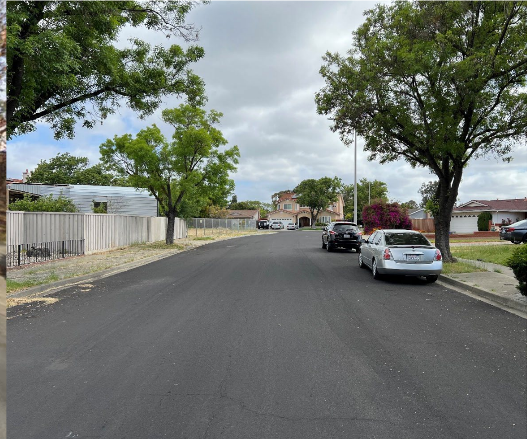
Figure 8: Guava Place After Patch Paving and Placement of Slurry Seal
