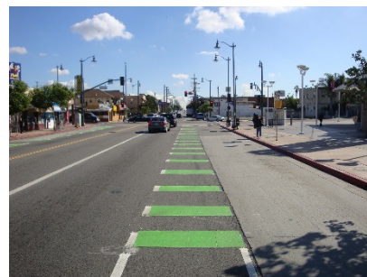
Green skip-striping at intersection where cars may merge across or into the bicycle lane
