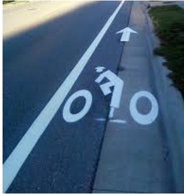
Bike lane painted over gutter pan
