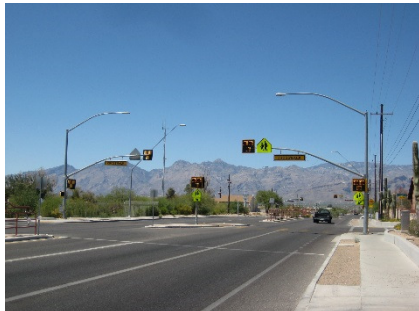
Pedestrian hybrid beacon at trail crossing
