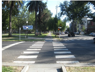
Stop bars and high-visibility striping at trail crossing
