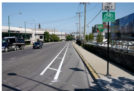
Buffered bike lane with wayfinding signage
