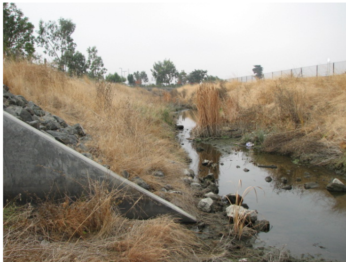
Figure 7: Line D at Area 3 Outfall
