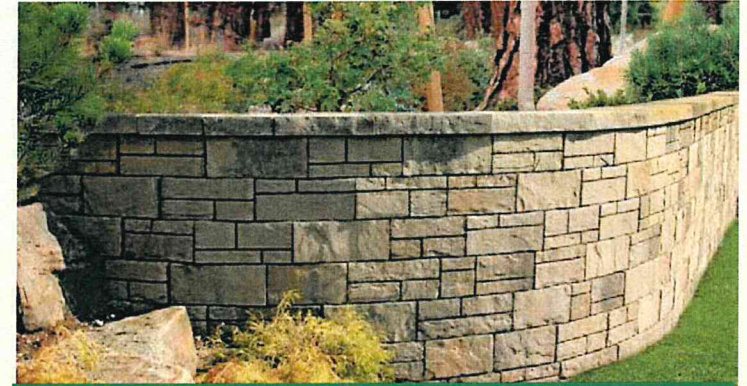
CMU RETAINING WALL
