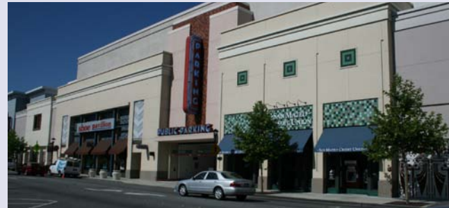
Parking should be located in the center of a block and visually de-emphasized from the street, as shown in this Redwood City parking structure.
