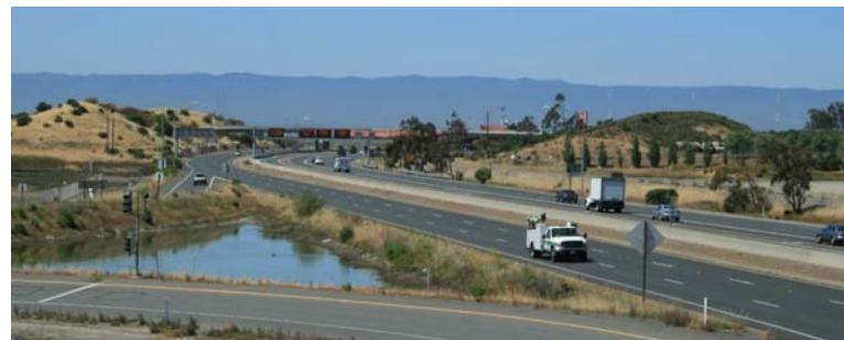
Highway 84 looking west toward the Dumbarton Bridge.
