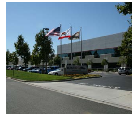
Thornton Business Center.
