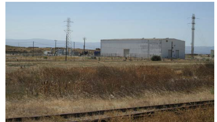
Vacant industrial lands in Area Two.
