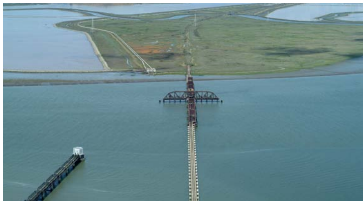
Aerial view of the Dumbarton Rail Bridge.
