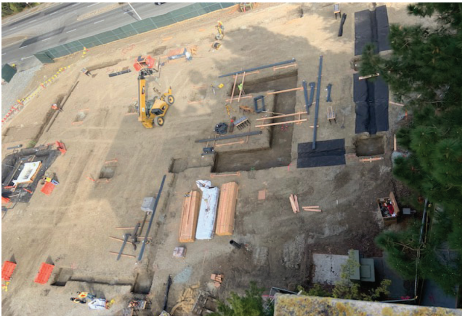
Foundation preparation at City Hall
