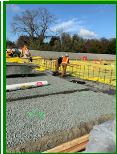
Figure 2: Concrete slabs are being poured for each of the new buildings.
