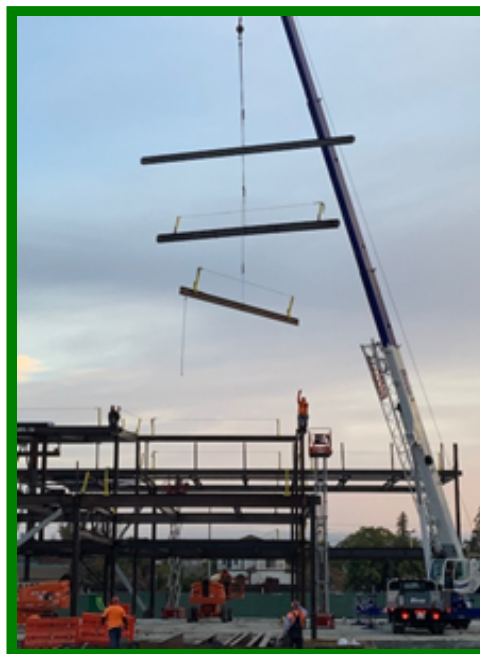
Figure 1: Steel erection began at the new City Hall on 01/21.
