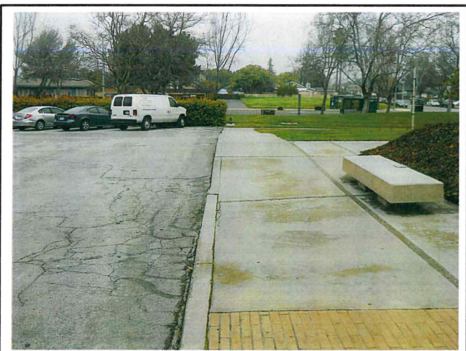
TP102 CITY ADMINISTRATION BUILDING New curb ramp for upgraded accessible parking
