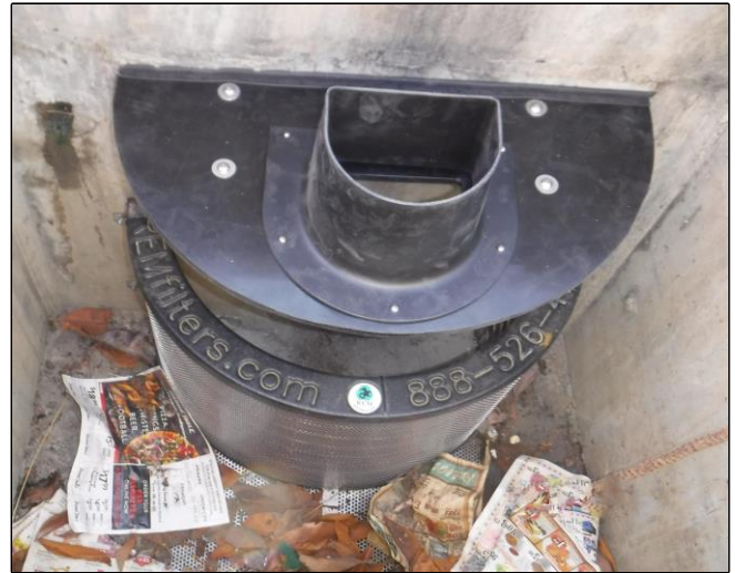
Standard REM CPS-PERF FTC device installation
