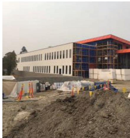
View of the library from the parking lot
