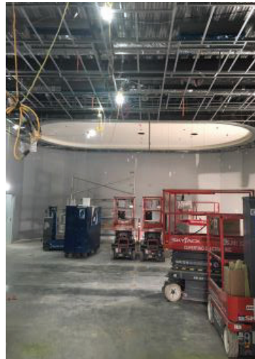
Raised ceiling above the City Council dais
