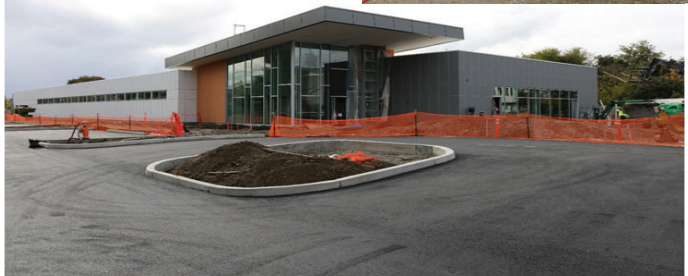
View of the police building from the parking lot
