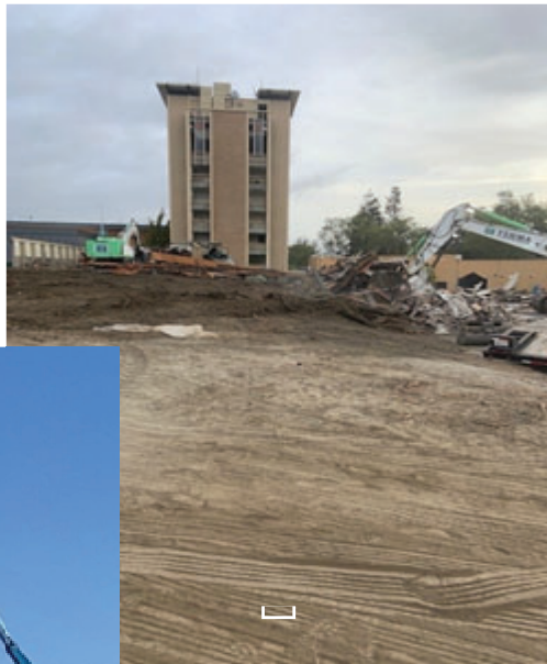
The tower minutes before demolition began.
