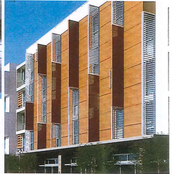
WOOD LOOK PANELS - THE QUAD, SAN MARCOS
