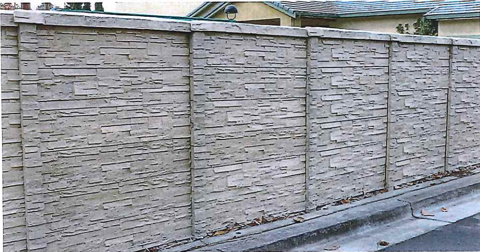
EXISTING 6' PRECAST CONCRETE FENCE
